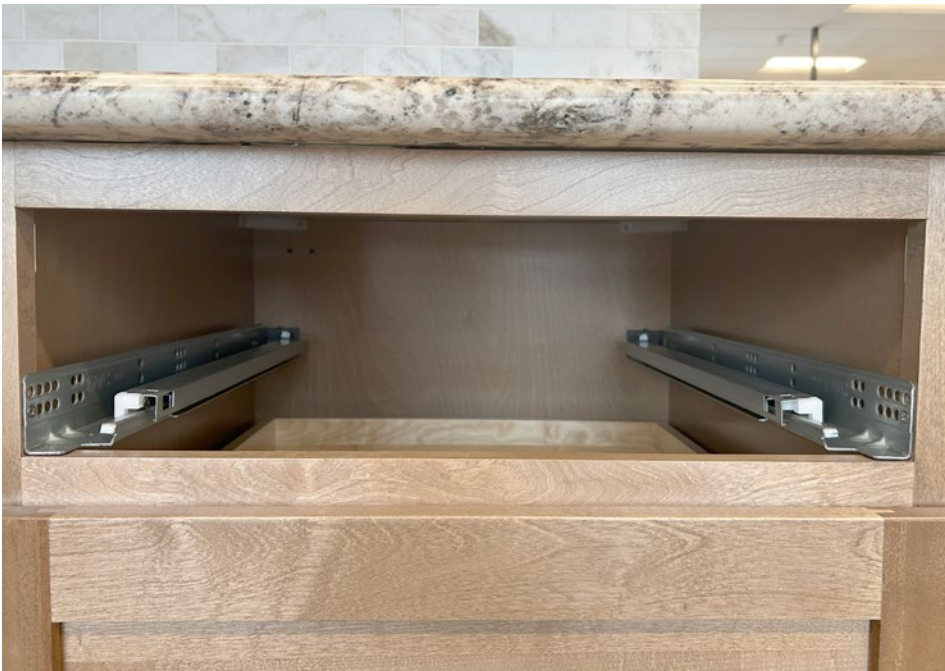
DRAWER SLIDE INSTALLATION
