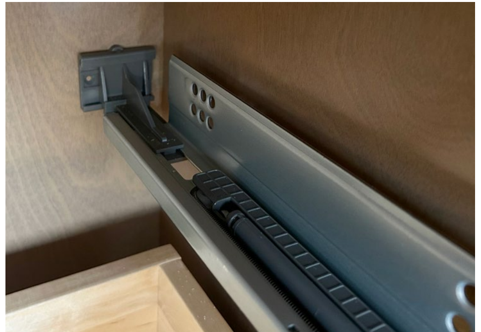
DRAWER SLIDE INSTALLATION
